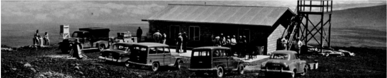
The observatory building in June 1956.
