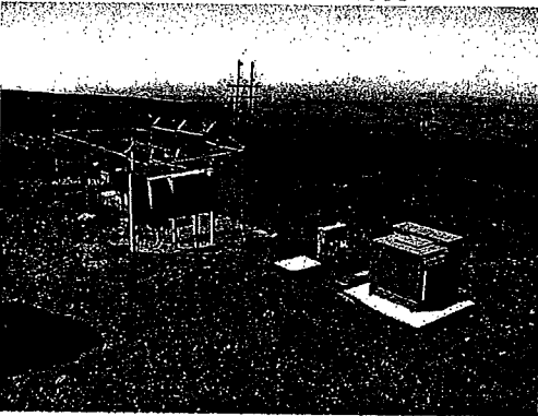
HECO OLD GENERATOR (CONSTRUCTED LATE 1967) HECO NEW GENERATOR CONSTRUCTED
