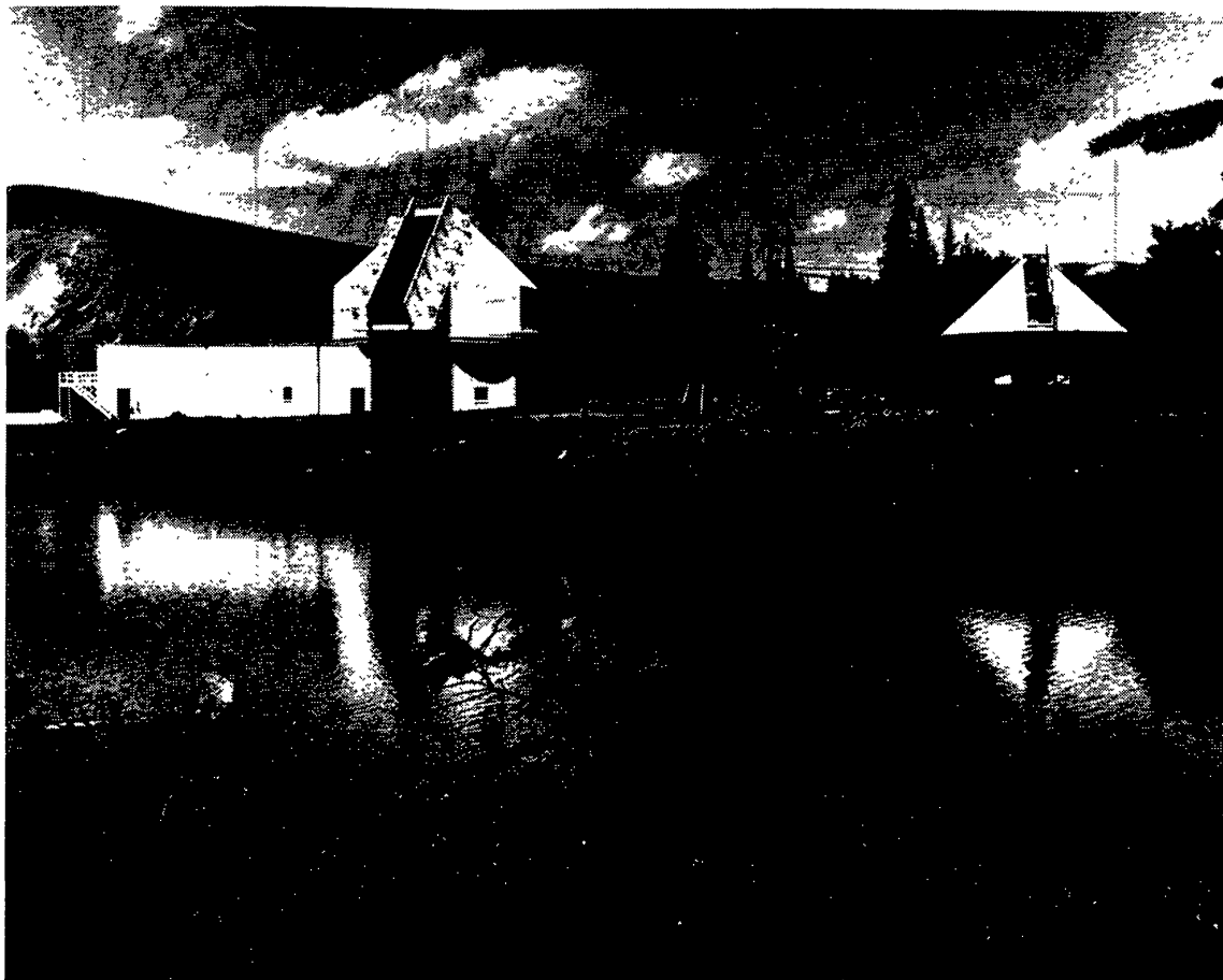
Fig. 1. The HAO Climax station is located at an altitude of 3394 m on the continental divide. The larger dome contains the 40-cm coronagraph-spectrograph and magnetograph. The smaller dome encloses the 13-cm coronagraph-spectrograph and flare patrol telescope. Snow covers the ground during much of the year and dictates the use of conical rather than the usual hemispherical domes.
