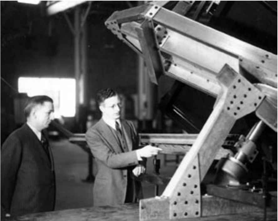
FIG. 4. Willard H. Dow (left) and Donald H. Menzel (right) inspect eclipse equipment made of lightweight "DowMetal", at the Dow Chemical Company in Midland, Michigan. This equipment travelled to Ak-Bulak as part of the Harvard-MIT expedition to the 19 June 1936 eclipse. Courtesy of Suzanne Menzel Synder and the Archives of the National Center for Atmospheric Research.
