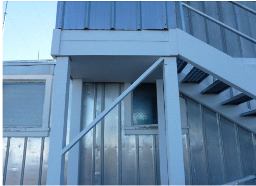
UCAR replaced structure holding up 'doghouse
